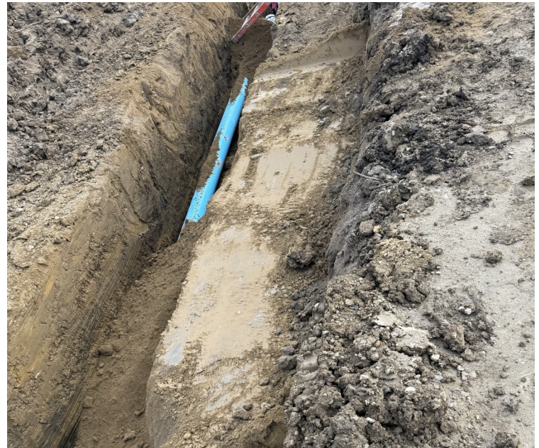
Domestic Water Piping to the Building
